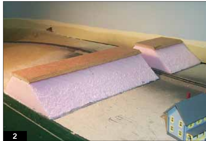
2 Fellow modeler Dave Montgomery and I started construction on the levee bridge by first cutting foam insulation board to represent the levee. The roadbed is made from a section of hardboard that has been beveled.
