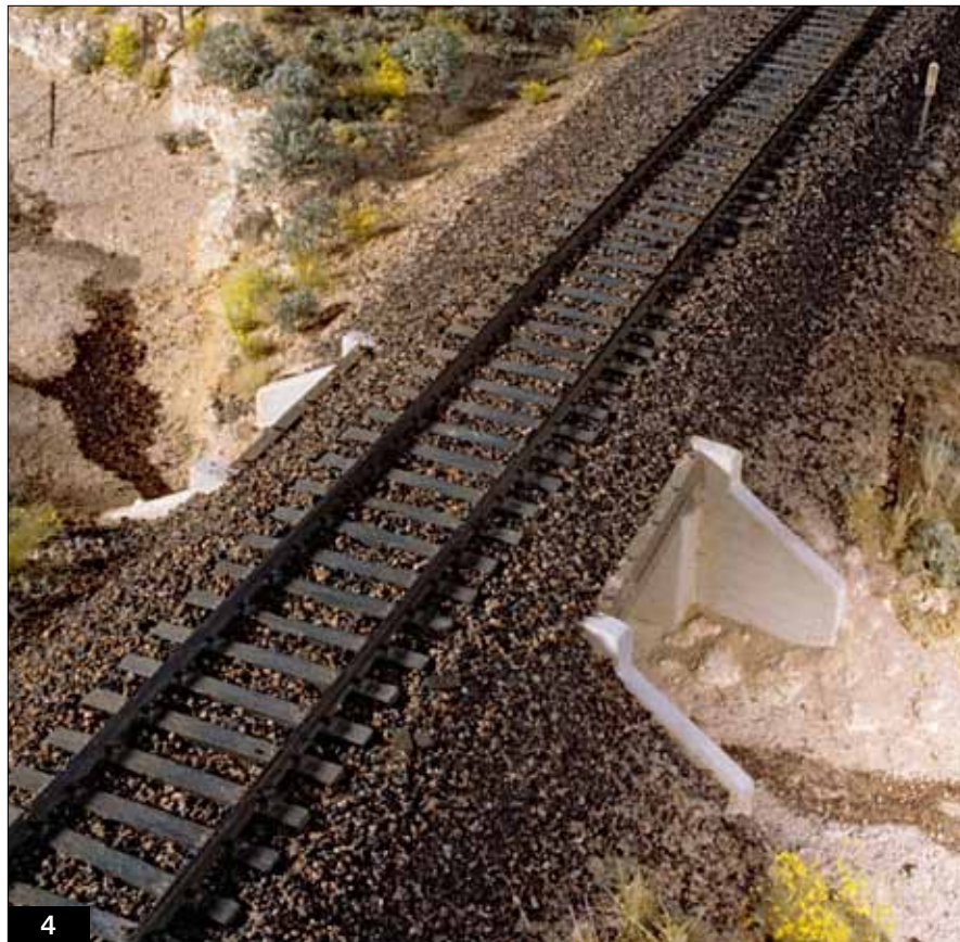
These bridges are identical to square culverts except they lack a floor. Desert ranchers employ water-wise mechanics of their own—note that the barbed wire fence is staked only at mid-channel. The other posts merely serve as wire spacers, allowing the fence to swing away in floods and shed debris.
