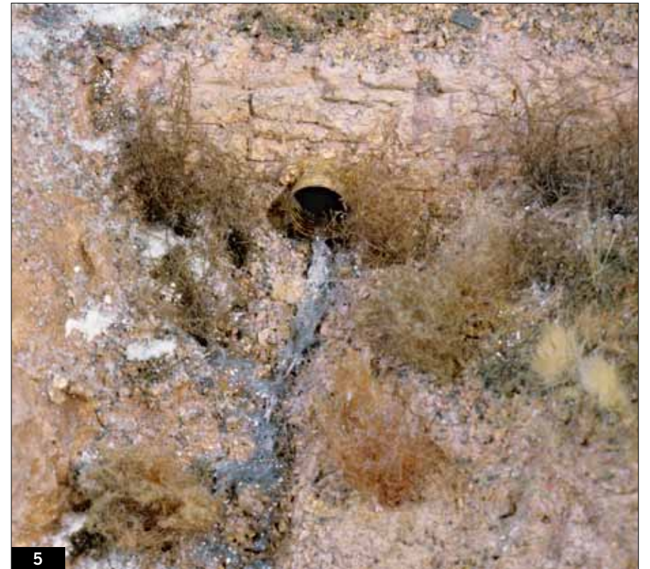
This 30" pipe culvert is typically found where trackside ditches converge into small streams. The spillway has been lined with riprap to prevent erosion.
