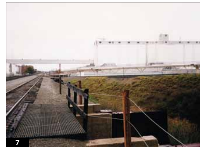
7 For the brown walkway, shown here on the prototype's flood gate (south) side, I cemented two HO scale running boards side-by-side and added styrene fence posts and railings.
